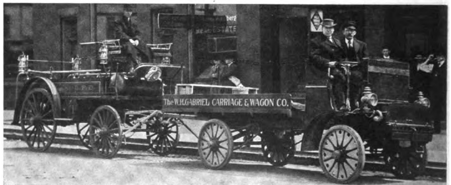
Grabowsky Power Wagon Delivers Lorain Hose Cart Over Roads
